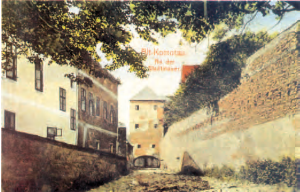
Fig. 10. The outer wall of inter-walls on the area along the Chomutovka by Riegerově street (based on Bret – Stiska – Pachner 1992)
