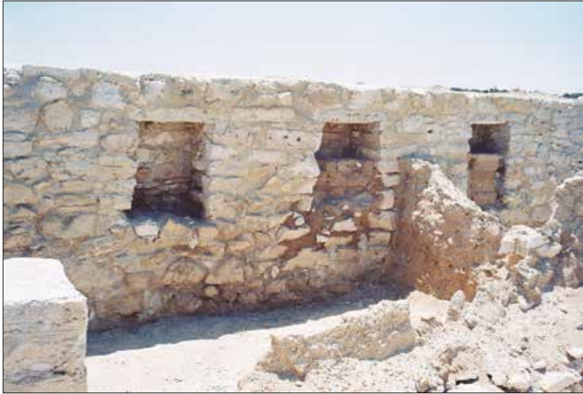
Fig. 6. Niches in the southern wall of Room 12a (photo by S. Medeksza).
