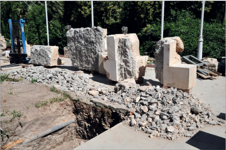
Fig. 3. The lion fragments in their new location in the gardens of the National Museum in Damascus: removing the old concrete backing of the statue, June 2017 (PCMA UW Documentation Center | photo B. Markowski)
