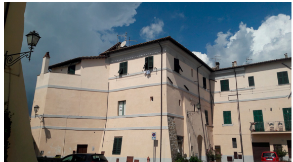
8. Palazzo Poniatowski as seen from the side of Piazza della Rocca – current state after destructions and remodelling, with several private flats inside
