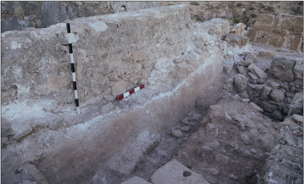
Fig. 18. Structure reinforcing the east wall of room D72 in trench D/T4, general view from the west (Photo M. Antos)
