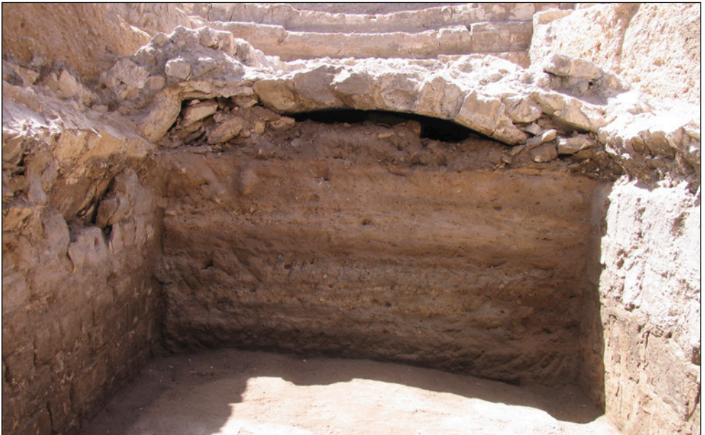
Fig. 13. Collapsed vault of the bath entrance chamber, view looking south (Photo G. Majcherek)
