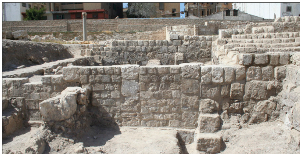
Fig. 24. North wall of vestibule R after restoration (Photo A. Piszczewski)
