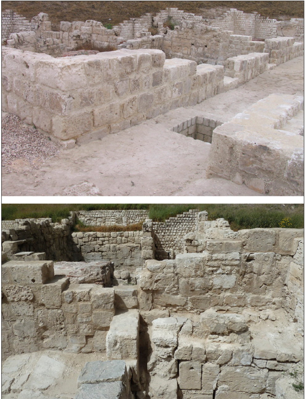
Fig. 19. Restoration in the domestic quarter: top, southwestern corner of building H after restoration; bottom, restored north wall of rooms H8a and H8b (Photos G. Majcherek, M. Polak)
