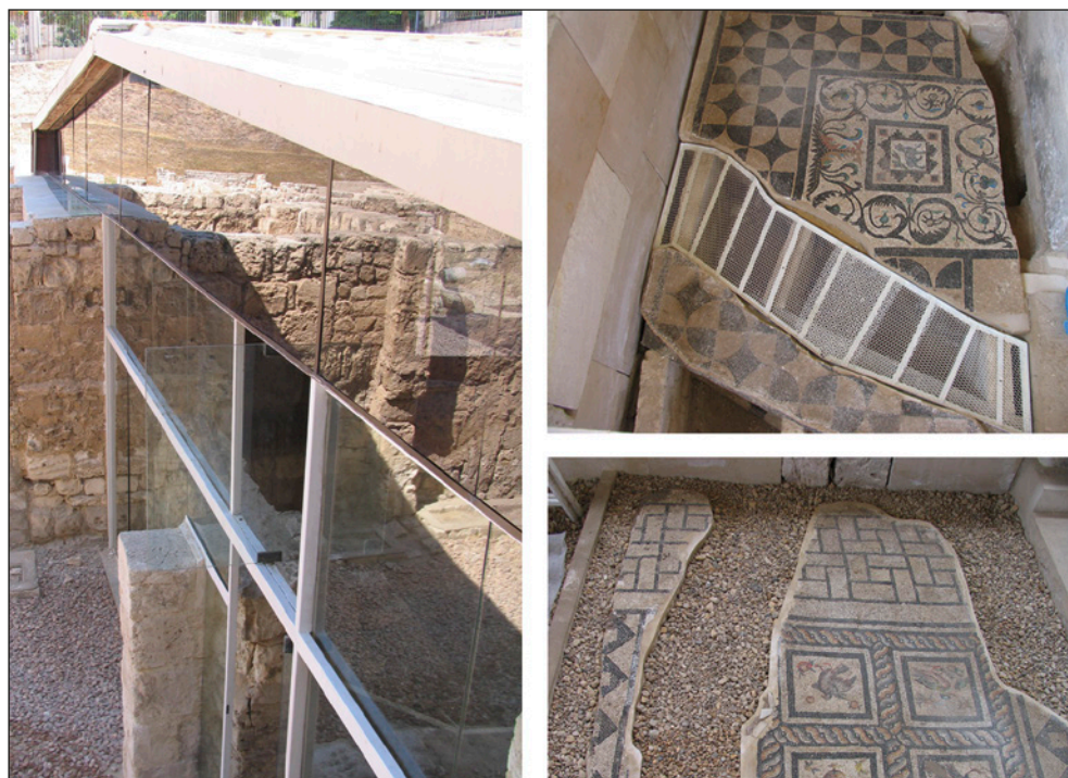
Fig. 17. Maintenance conservation in the Mosaic Shelter: left, repaired west glass wall; top right, ventilation grille around the mosaic with panther (α-6); bottom right, restored edges of the mosaic with birds (α-5) (Photos G. Majcherek)
