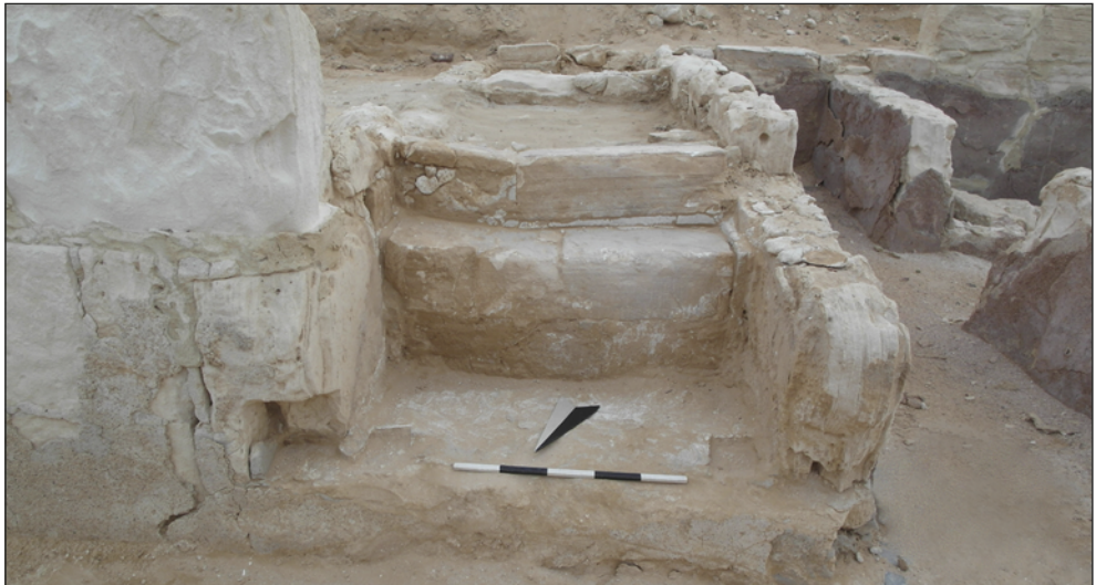
Fig. 9. Entrance and stairs 16 in the Southern Bath (Photo R. Czerner)
