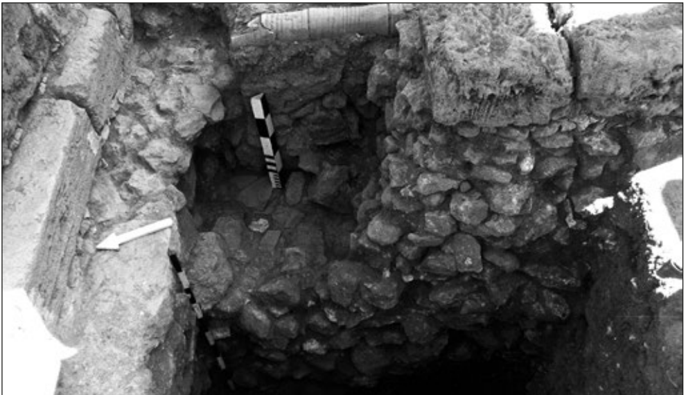
Fig. 18. Foundation of the eastern stylobate at its northern end (excavated in 1993) (PCMA Nea Paphos project/photo W.A. Daszewski)
