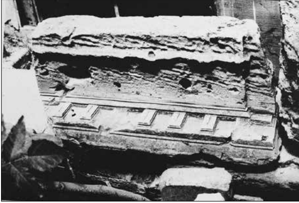
Fig. 9. Marina el-Alamein, houses in the southern area of the town, cornice with flat grooved ( a travicello ) modillions and a smooth frieze (photo by P. Pensabene).
