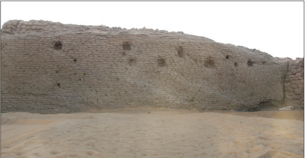
Fig. 3. Facing of dried brick between the towers NE and N.2 (Photo W. Godlewski, PCMA UW)
