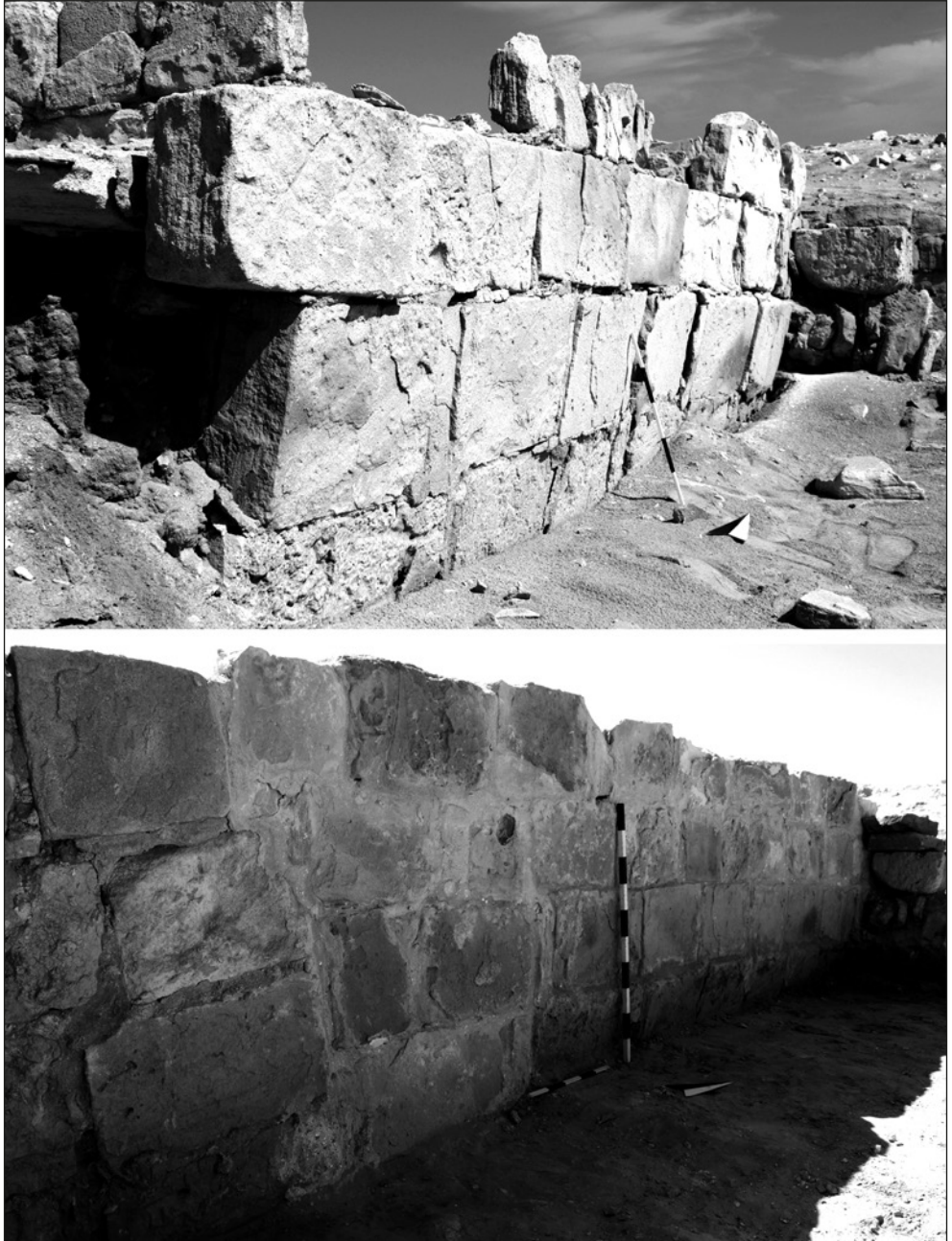
Fig. 3. Houses H2 and H2a: retaining wall before (top) and after (bottom) conservation in 2012 (Photos R. Czerner)
