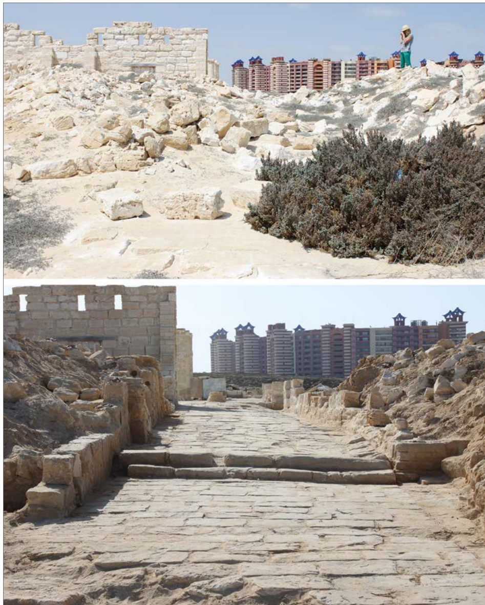
Fig. 6. Street east of the forum, view from the east: top, before cleaning and preservation; bottom, after cleaning and preservation in 2017 (Polish–Egyptian Conservation Mission Marina el-Alamein/ photos R. Czermer)
