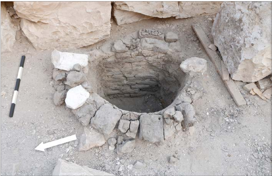
Fig. 3. Southeastern foundation pit after investigation, viewed from the west (IFAO/PCMA UW/photo M. Caban)
