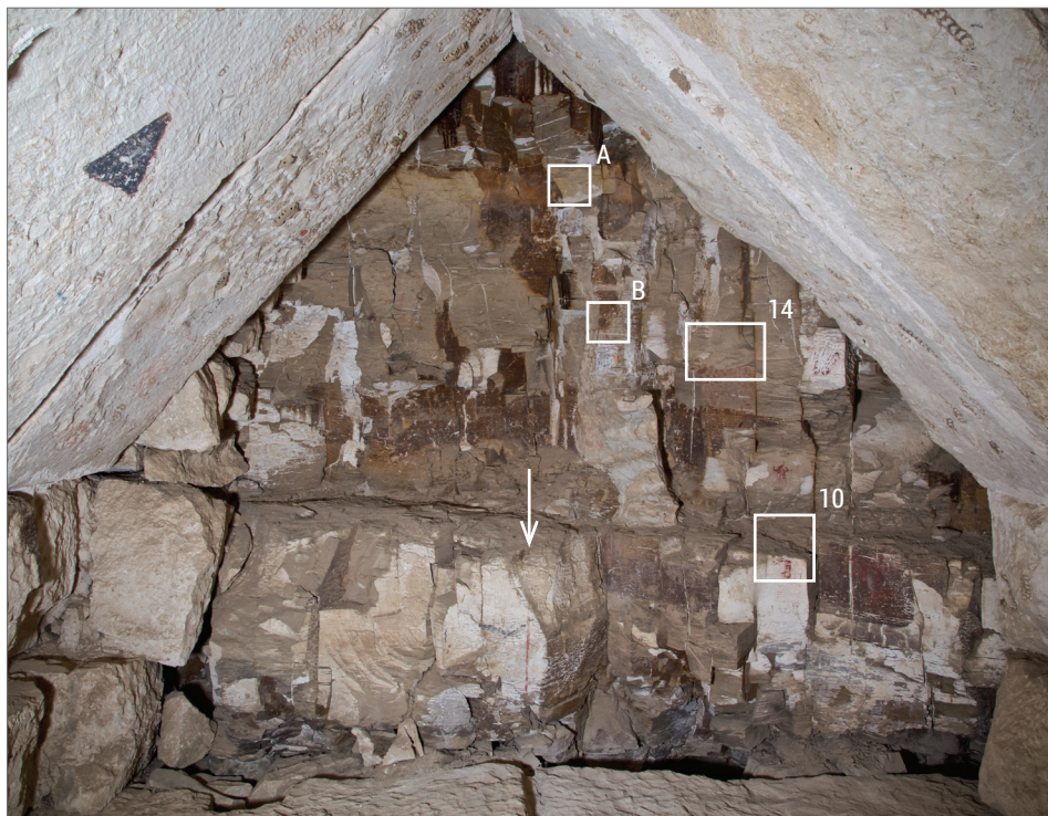
Fig. 5. Location of dipinti on the rock-cut west wall of the relieving chamber above the Bark Hall; arrow indicates the line of symmetry (PCMA UW Temple of Hatshepsut Project/photo M. Jawornicki)
