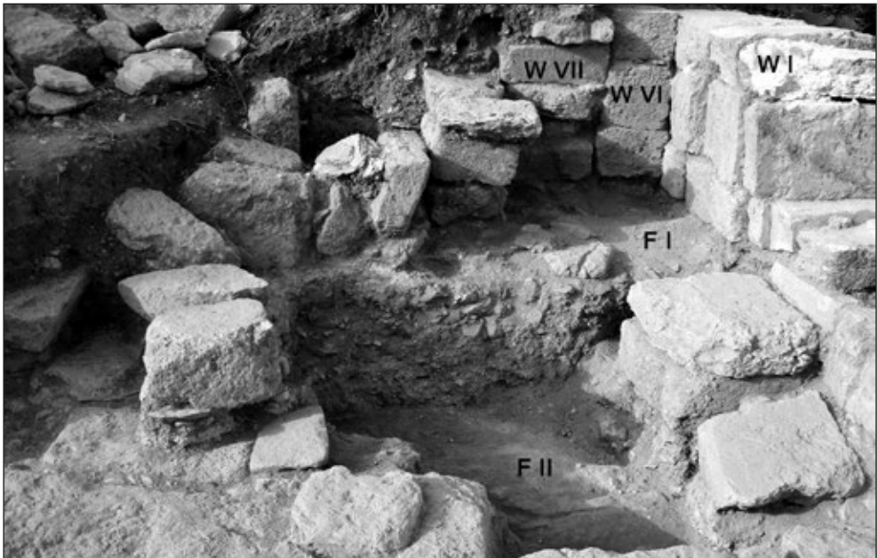
Fig. 6. Two successive floor levels: F I (background) and F II (foreground), W I to the right, view facing south (PCMA Beit Ras Project/photo J. Młynarczyk)
