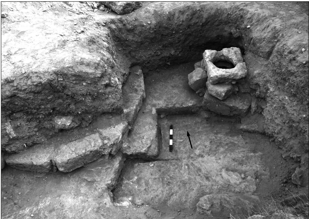
Fig. 22. Cistern framing (Loc. 006) in Area 1-S, Sq.9 on bedrock with traces of the original stone quarrying; note the semicircular line of W IV to the left; view facing north (PCMA Beit Ras Project/photo D. Mazanek)
