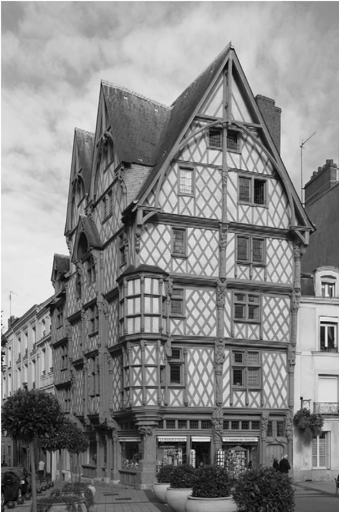
Photo 2. Maison d' Adam , Angers, France – renovation in 1994
