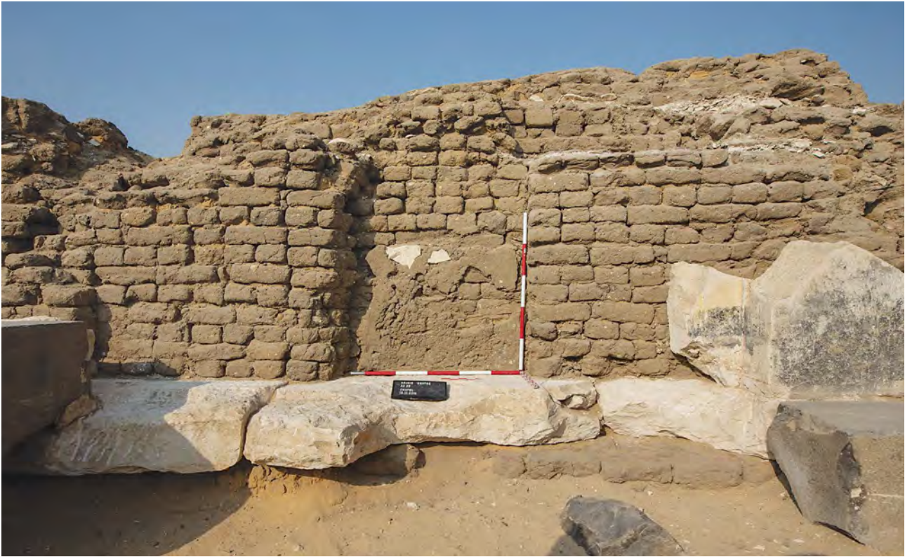
Fig. 5 Western wall in Chapel 1 (photo P. Košárek)
