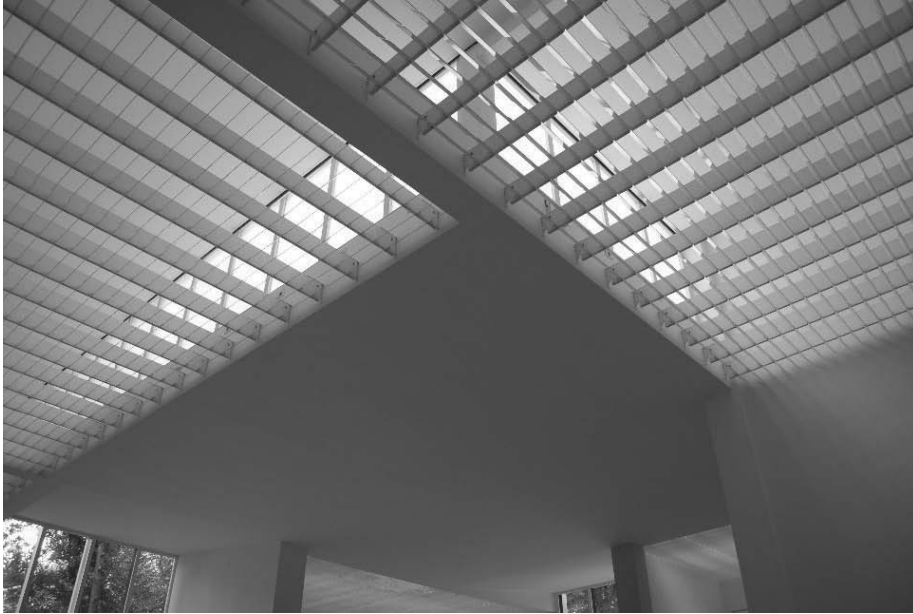
Illustration 2. Interior of the Netherlands Pavilion on the Venice Biennale grounds, arch. Thomas Gerrit Rietveld, 1953
