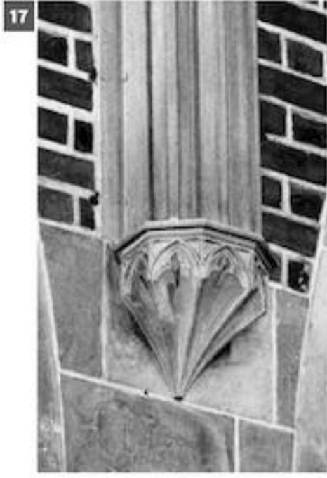
17. Kraków cathedral, corbel on the northern wall of the choir. Photo by Piotr Pajor. → see p. 17
