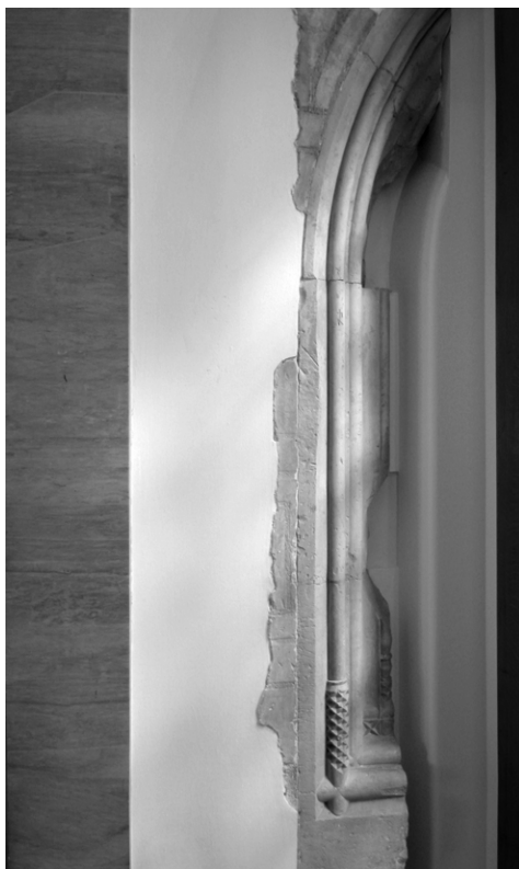
FIG. 7: Prague Castle, the former palace of Archduke Ferdinand by the White Tower. Part of a window (or door) on the eastern end of the palace's northern facade on the first-floor level (© Petr Chotěbor).
