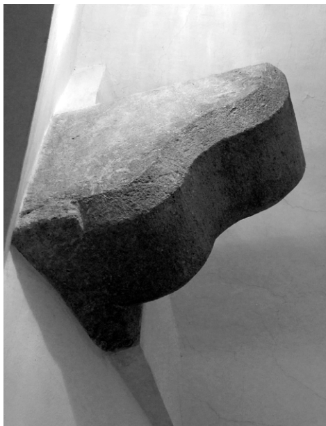
FIG. 6: Prague Castle, the former palace of Archduke Ferdinand by the White Tower. Corbel of the oriel that used to be on the first floor on the western end of the palace's southern facade (© Petr Uličný).
