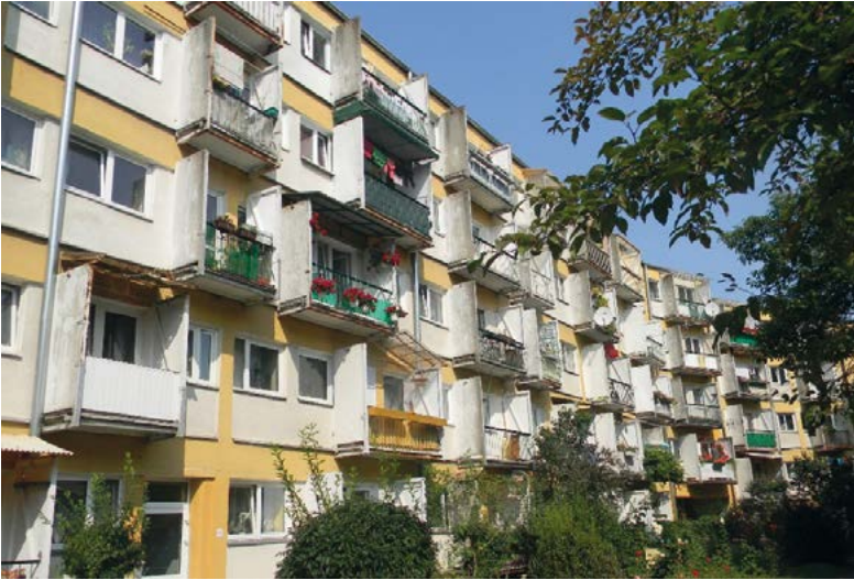
Figure 2. Observed “serpentine” building. Photo: Natalia Otrishchenko (2018)
