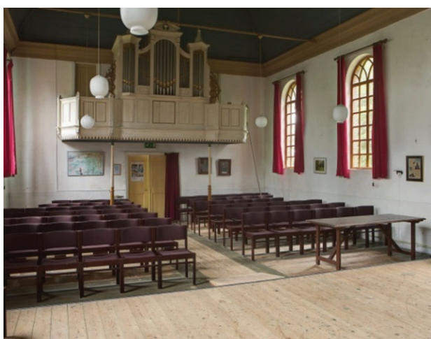
Fig. 4. View of the interior of the former church in Klein Wetsinge towards the porch. Condition before renovation, 2011 (source: [20])
