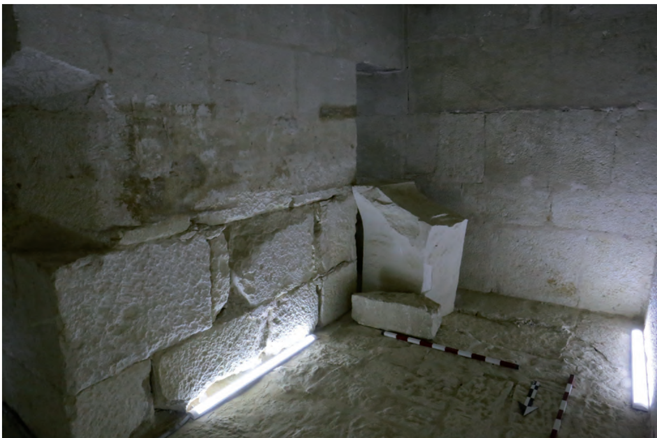
Fig. 8 East wall of the burial chamber showing the outline of the sarcophagus, the corner of which is preserved in situ ; most of the floor is reconstructed. The upper part of the entrance shows the adjustment that facilitated manipulation of the coffin during burial (photo H. Vymazalová)
