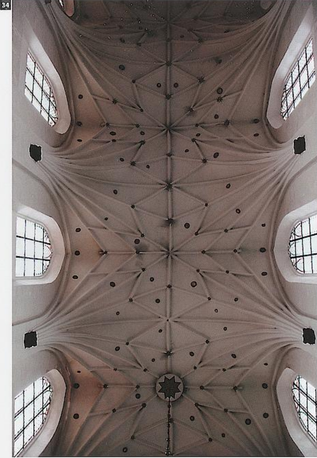
34. Oliwa, Cistercian Church, vault of the nave. Photo: author
