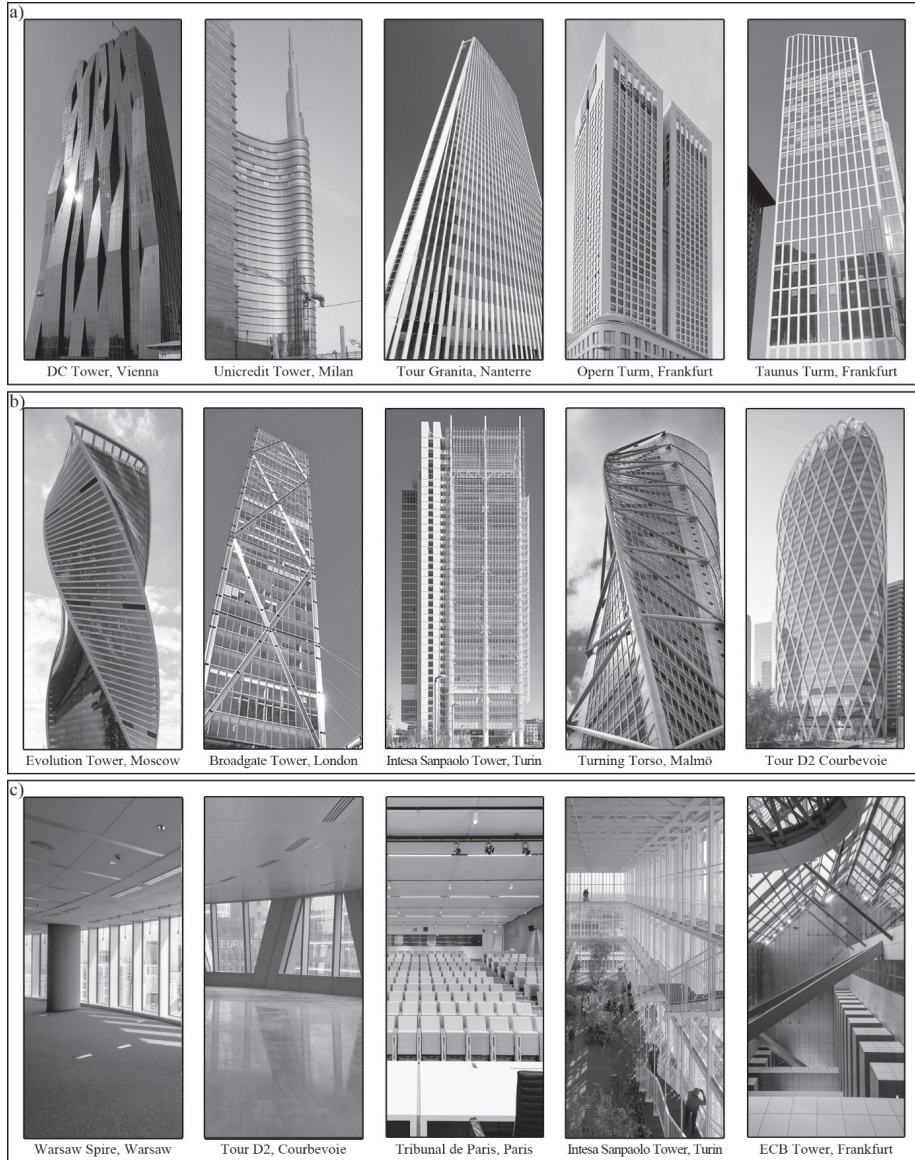
Illustration 2. Load-bearing structure and the aesthetic expression of a high-rise building: a) different design of elevations with “hidden” load-bearing structure; b) elevations with the load-bearing structure exposed; c) interiors with exposed load-bearing structure
