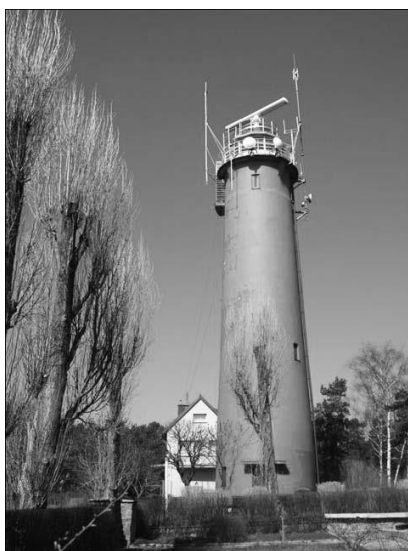
Fig. 2. The Krynica Morska lighthouse, a present-day view Source: Author's collection
