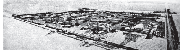
Fig. 9. The prospect of a quarter-complex in Makeevka (arch. M. Stam, early 1930s) (source: [20])
