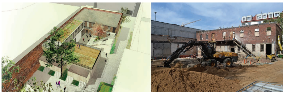
Figure 4. Local Activity Center, Prądyńskiego 39a. Project and work progress 21/09/2018
