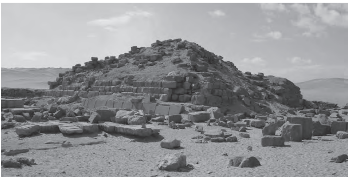
Fig. 3 The current remains of the “pedestal building” viewed from the north-east (photo M. Nuzzolo)
