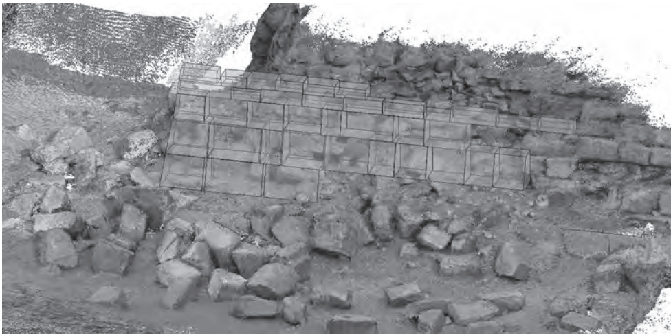
Fig. 8b Schematic reconstruction of the south-western corner of the “pedestal building” (elaboration in BIM by P. Zanfagna, based on laser scanner and photogrammetric data)
