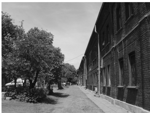
Photo 1. Historic workers' estate at Księży Młyn – western elevation of houses at Przędzalniana Street
