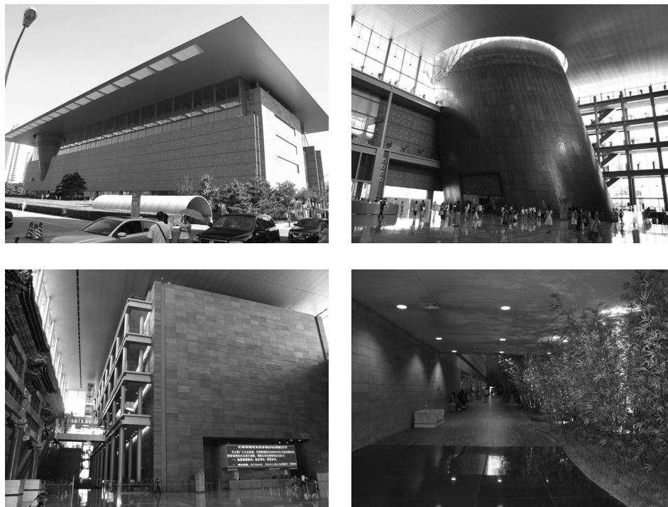
Fig. 2. Cui Kai (CAG Design Studio), Jean-Marie Duthilleul and Etienne Tricaud (studio AREP), Capital Museum, Beijing (Chaoyang District) 2006, (photo J. Kucharzewska, 2009). A-outside view; B-Oval Exhibition Hall, C-Rectangular Exhibition Hall; D – basement story
