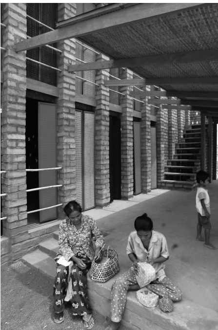
Fig. 5. Openings left between bricks providing natural ventilation. Image by courtesy of Architects Rudanko + Kankkunen
