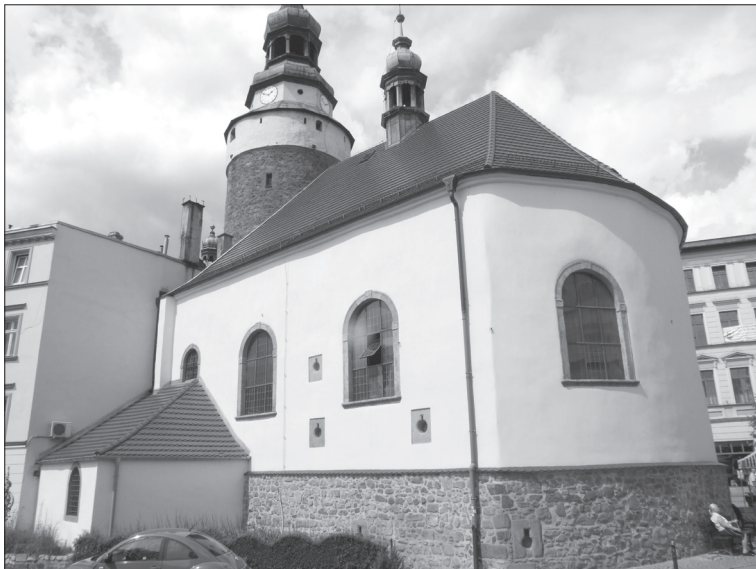
Figure 4. Hirschberg, St. Ann's Chapel, former bastei
