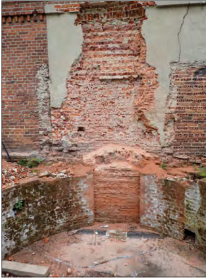
Fig. 9. The Konsum building. The northern elevation of the one-storey part with the remains of the ice house wall. A view from the north as of the summer of 2020, photograph by J. Pietrzak
