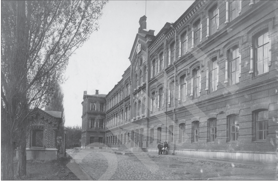
5. The main building of Kharkiv Institute of Technology, 1900s (materials of the Museum of National Technical University “Kharkiv Polytechnic Institute”)
