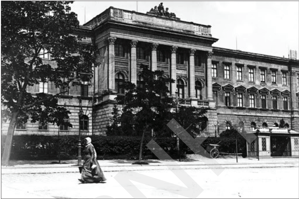
3. Main building of Lviv Polytechnic built by Julian Zachariewicz in 1877. The photo from free sources – https://photo-lviv.in.ua/lvivska-politehnika-na-45-chorno-bilyh-foto-1900-1939-rokiv/
