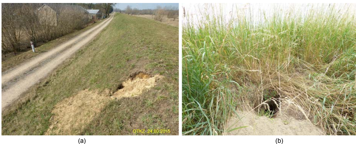
Figure 1. Presents damaged flood banks caused by animals. The holes were caused by the beavers living in the area. Grazing animals on the levees and in their immediate vicinity violates the construction of levees and causes changes in soil mass. Photo by Janusz Orzepowski
