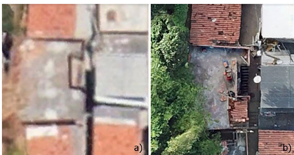
Fig. 9. Google Earth a and drone b. Unprotected stairways and slabs became visible.
