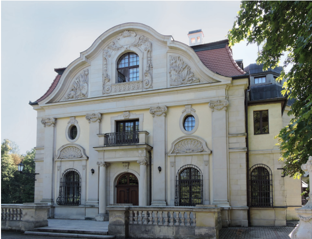
Fig. 3. Palace in Smolice. North-eastern elevation of the main body of the palace (arch. “Gaze & Böttcher”, photo by E. Grochowska/K. Stefański, 2019)
