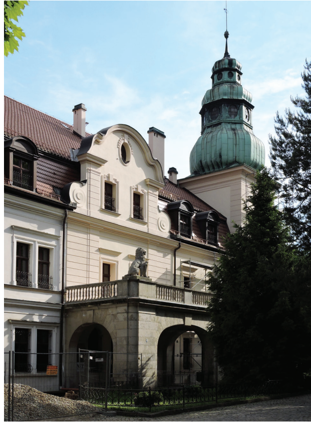
Fig. 12. Palace in Kamieniec (Kaminietz) near Tarnowskie Góry – façade. Restructuring by „Gaze & Böttcher”, 1910 (photo by E. Grochowska/K. Stefański, 2021)
