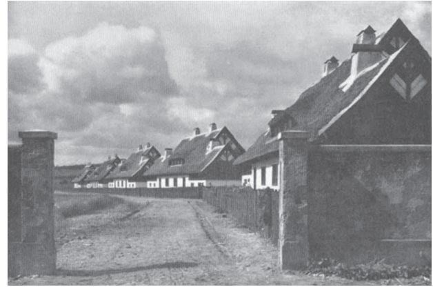
Fig. 2. Semi-detached houses of Schlesische Heimstätte , the settlement for policemen designed by Ernst May, Prudnik (formerly Neustadt), 1922–1923 (source: [21, p. 152])
