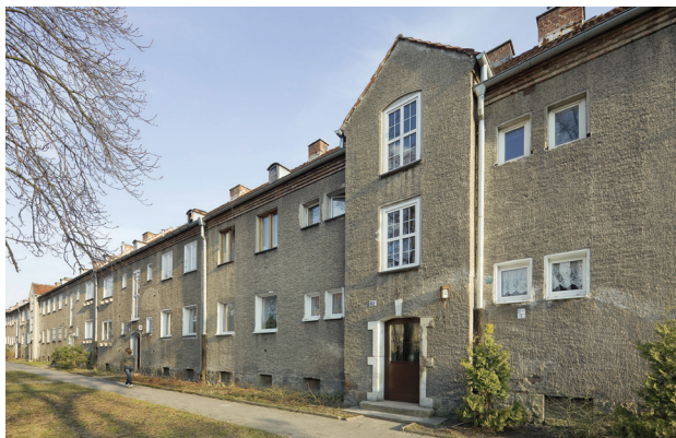
Fig. 9. Multifamily house of Schlesische Heimstätte , designed by Franz Auer and Herbert Wiehr, Wrocław-Psie Pole (formerly Breslau-Hundsfield), Piwnika-Ponurego Street (formerly Dreyse Strasse, Hofmann Strasse), 1940–1943 (photo by S. Klimek)
