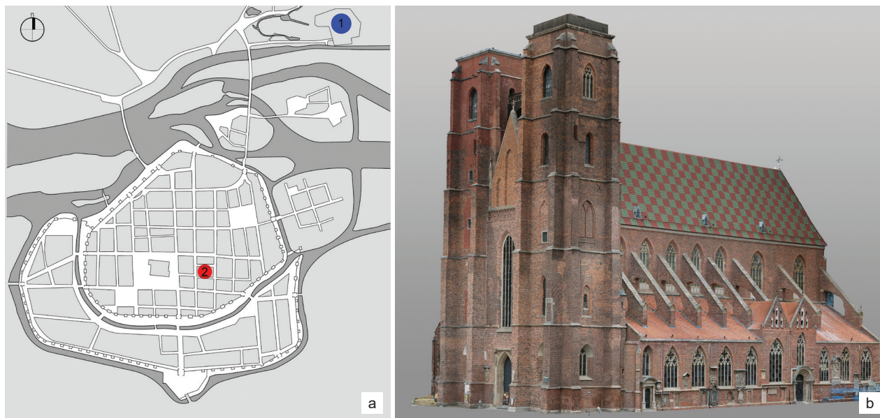
Fig. 1. Wrocław. Relocation of the portal from Ołbin.
