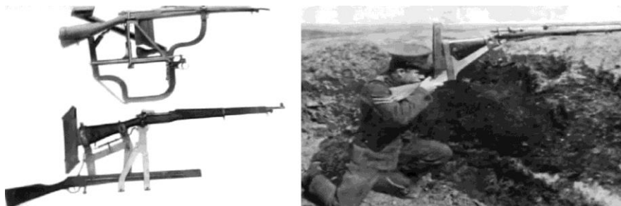
Fig. 11. Special designs facilitating shooting from behind a cover during WW I.
