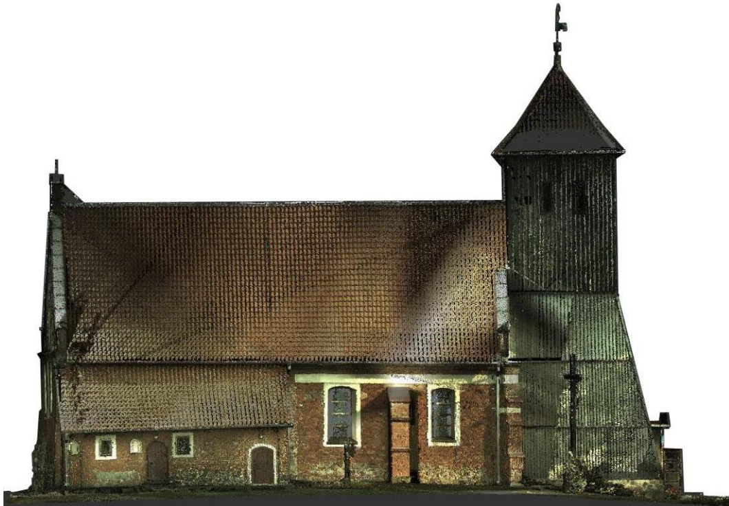
Fig. 1. North elevation of the church in the form of a point cloud with the superimposed photos Source: Own work.
