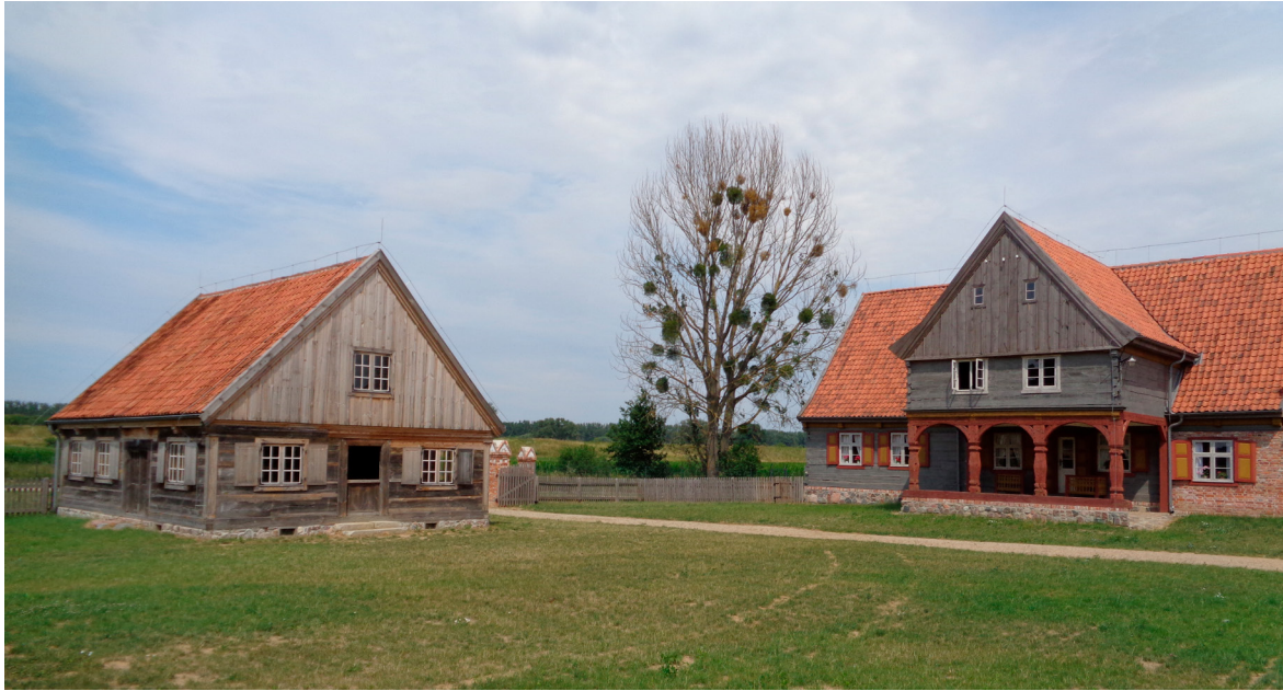
11. Farmhands' cottage from Mątownskie Pastwiska (1827) and the residential section of the Kaniczki homestead (1757), Olender Ethnographic Park in Wielka Nieszawka, 2018
