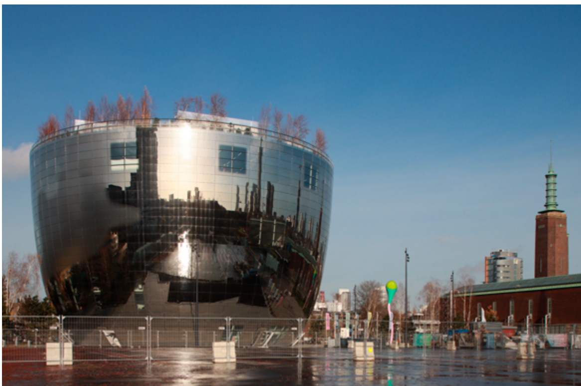
1. Depot, Rotterdam: general view, Photo Tomasz Zaucha, 2021
