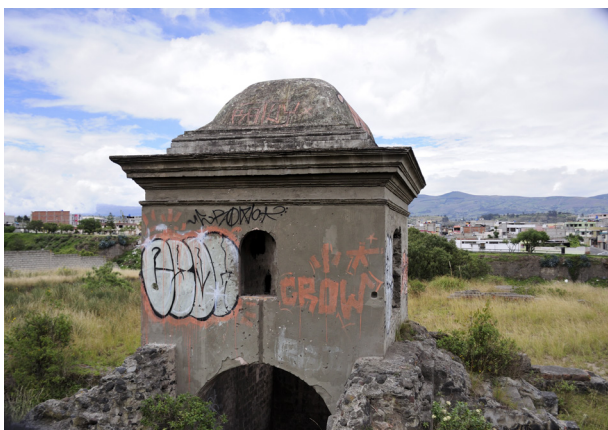
Figure 2. Latacunga – the old San Gabriel textile mill, located in the river valley and so inundated by mudslides following the 1877 eruption of Cotopaxi
