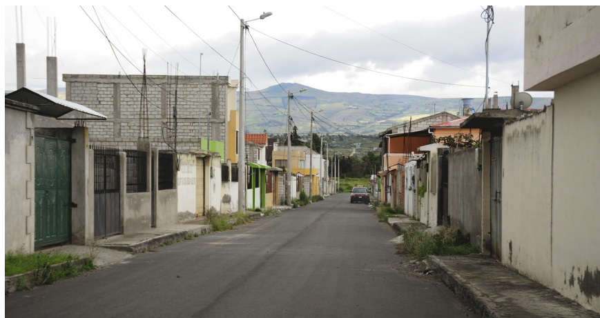
Figures 7. New housing construction in Nueva Vida/Campo Verde (Latacunga) Photo taken by: Mirosława Czerny
