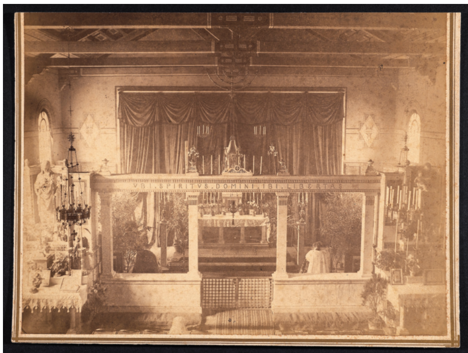
Fig. 5. Church of the Resurrection of the Lord in Cracow. Interior view towards the altar wall with visible partition.
