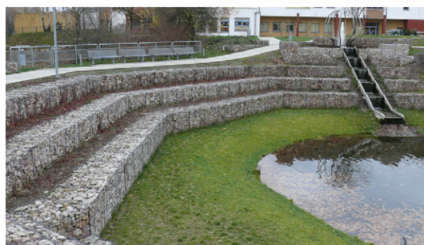
Fig. 11. Gabions - decorative reinforcement (built of rock fragments) of the slopes of the so-called "pits", i.e. former „Count's clay pit ponds". Photo by M. Górska-Zabielska (2015).
