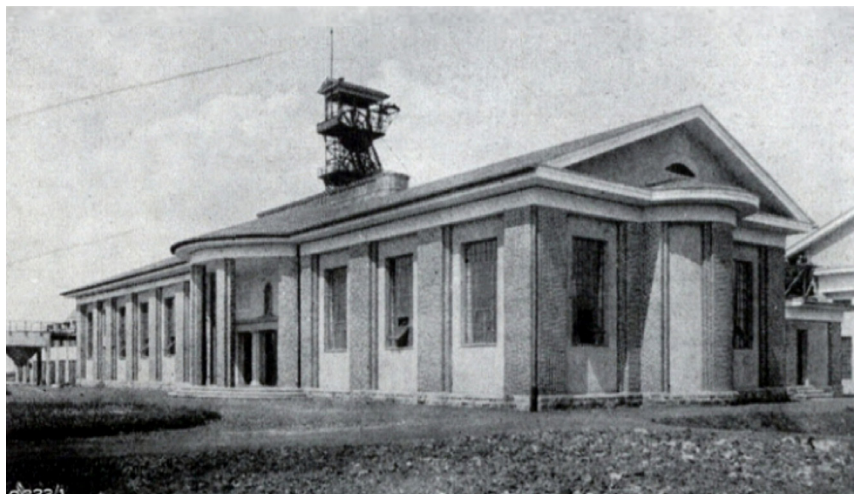
Photo No. 1. The pithead building of "Graf Franz" coal mine
