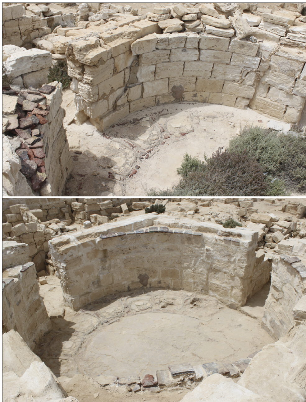
Fig. 2. The tholos of the Northern Bath before and after conservation in 2014; note the bricks of the base of the dome over the chamber [see also above, Fig. 11 on page 181] (Photos R. Czerner)
