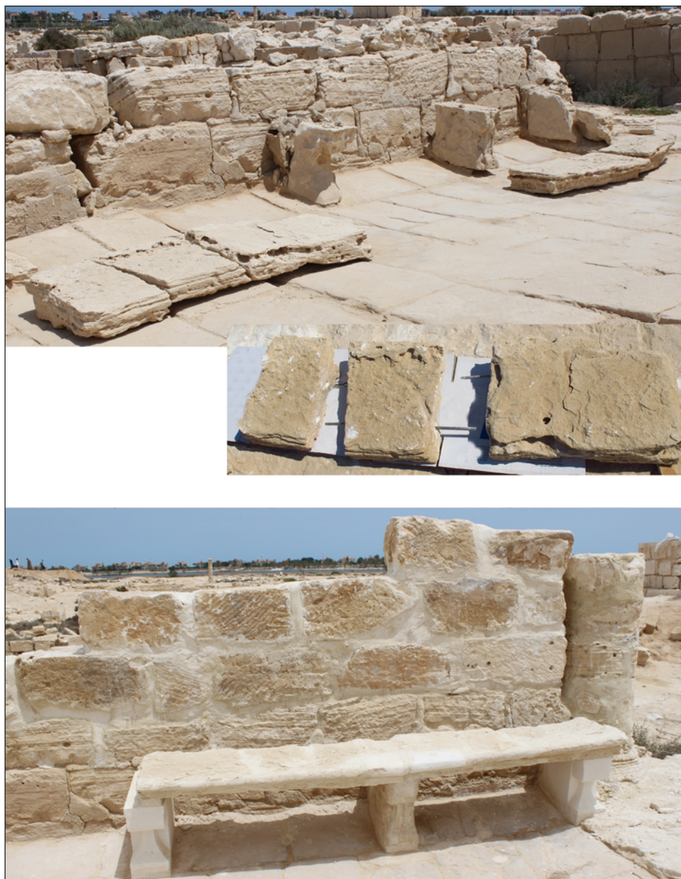
Fig. 1. Conservation of bench seats against the north wall of the central square: top, before conservation; center, conservation in progress; bottom, after conservation in 2014 (Photos R. Czerner, P. Zambrzycki)
