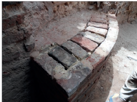
Fig. 10. Preserving the furnace in the destrictarium of the baths (PCMA UW Alexandria Kom el-Dikka Project | photo G. Majcherek)
