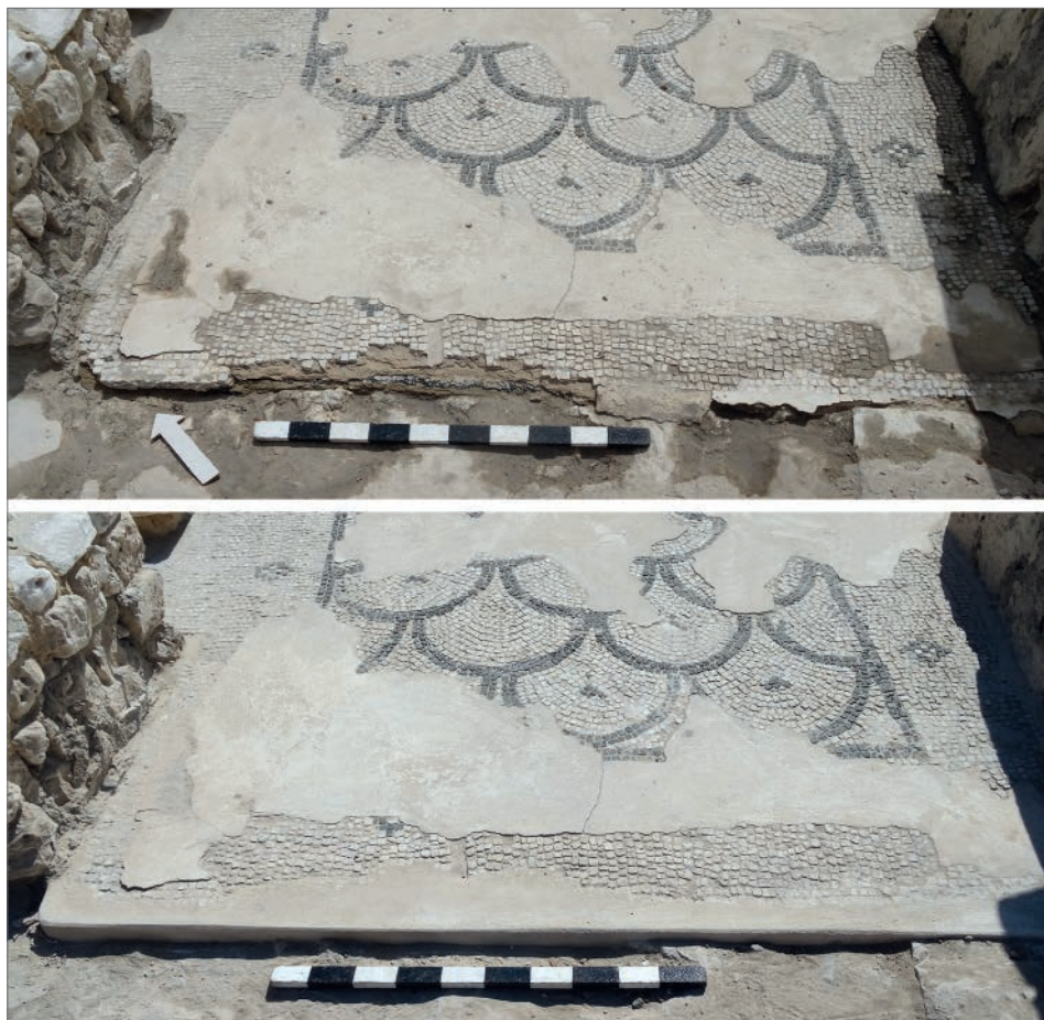
Fig. 15. Damaged mosaic in the northern vestibule of the theatre: top, before repairs and bottom, following preservation (PCMA UW Alexandria Kom el-Dikka Project | photos G. Majcherek)
