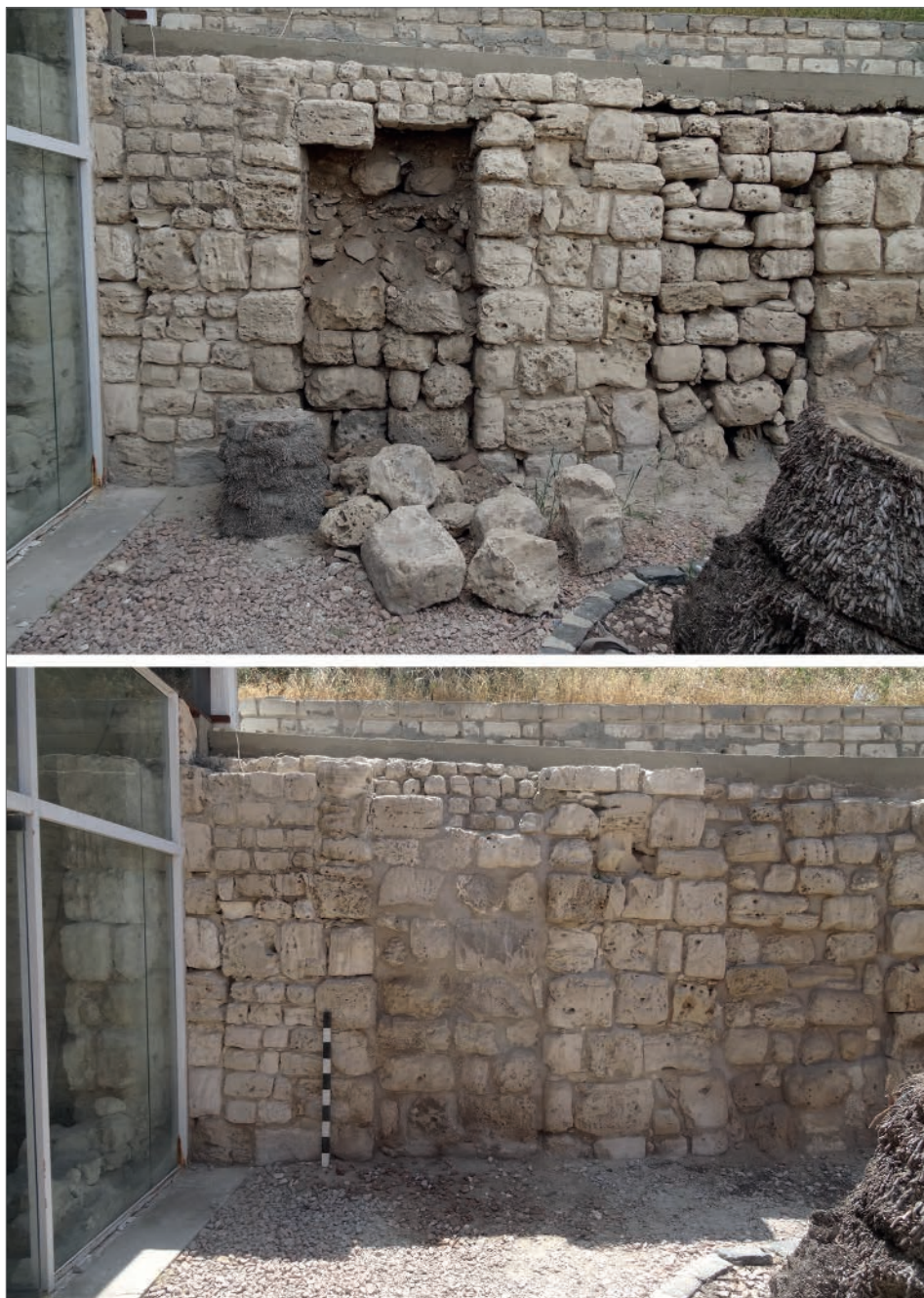
Fig. 13. Walled doors in rooms E-2 and E-4: top, prior to the preservation in 2018 and, bottom, after preservation (PCMA UW Alexandria Kom el-Dikka Project | photos G. Majcherek)
